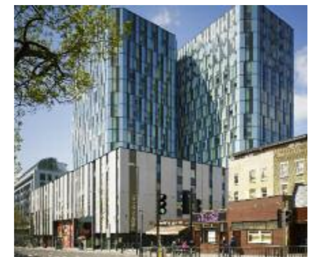
FAR LEFT: New, flexible workspace - 'White Collar factories' and LEFT: existing offices converted to student housing at King's Cross (AHMM)
