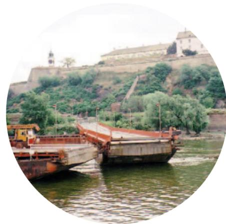
Left: It took 60 days to install this temporary barge bridge across the river Danube at Novi Sad. At 9pm every evening a central section opened up to allow river traffic to pass.
