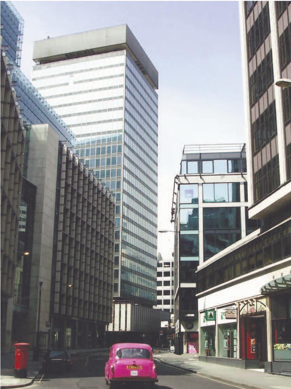
olition and the completion of the new building last year? Thereby hangs a fascinating tale – no pun intended. What pun? you might ask – the answer to which lies in the unusual construction of the Kleinwort Benson building as a column-free office tower with a central concrete core (constructed using an early slip-form method) whose floors are suspended on perimeter hangers carried by a large concrete 'umbrella' cantilever at the top.
