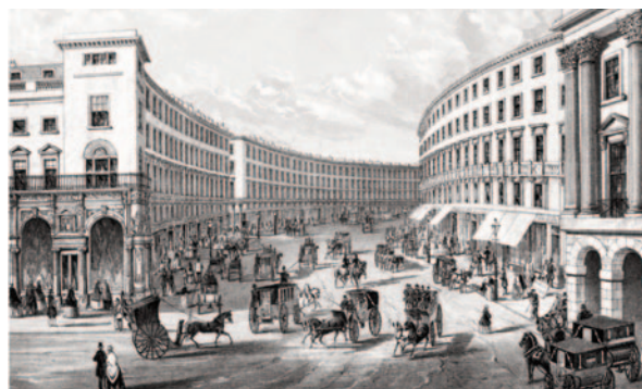
6 John Nash's stucco terraces, Regent Street, demolished 1895-1927.
