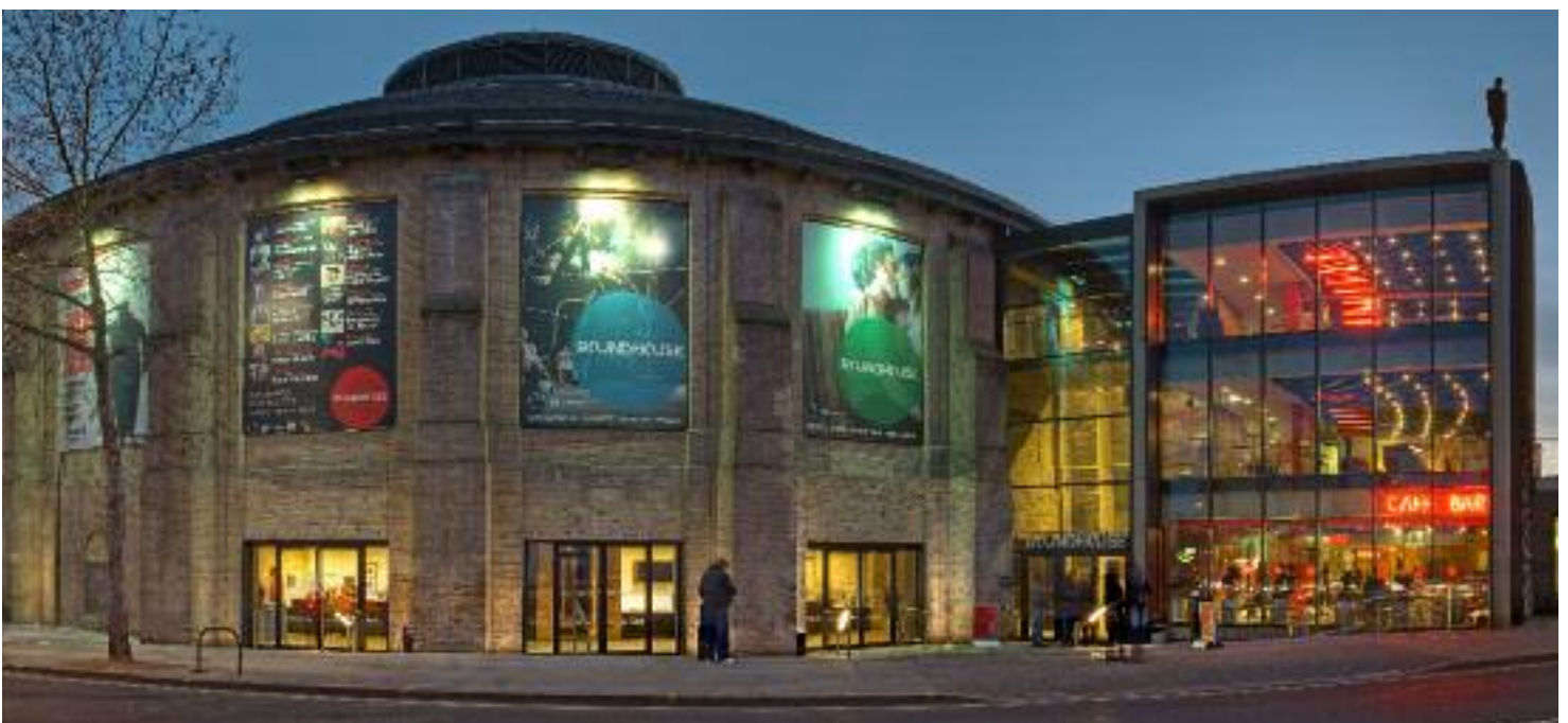
The Roundhouse Theatre is one of the most significant buildings in Camden and winner of the best project five years' on category. Photo Will Pearson
