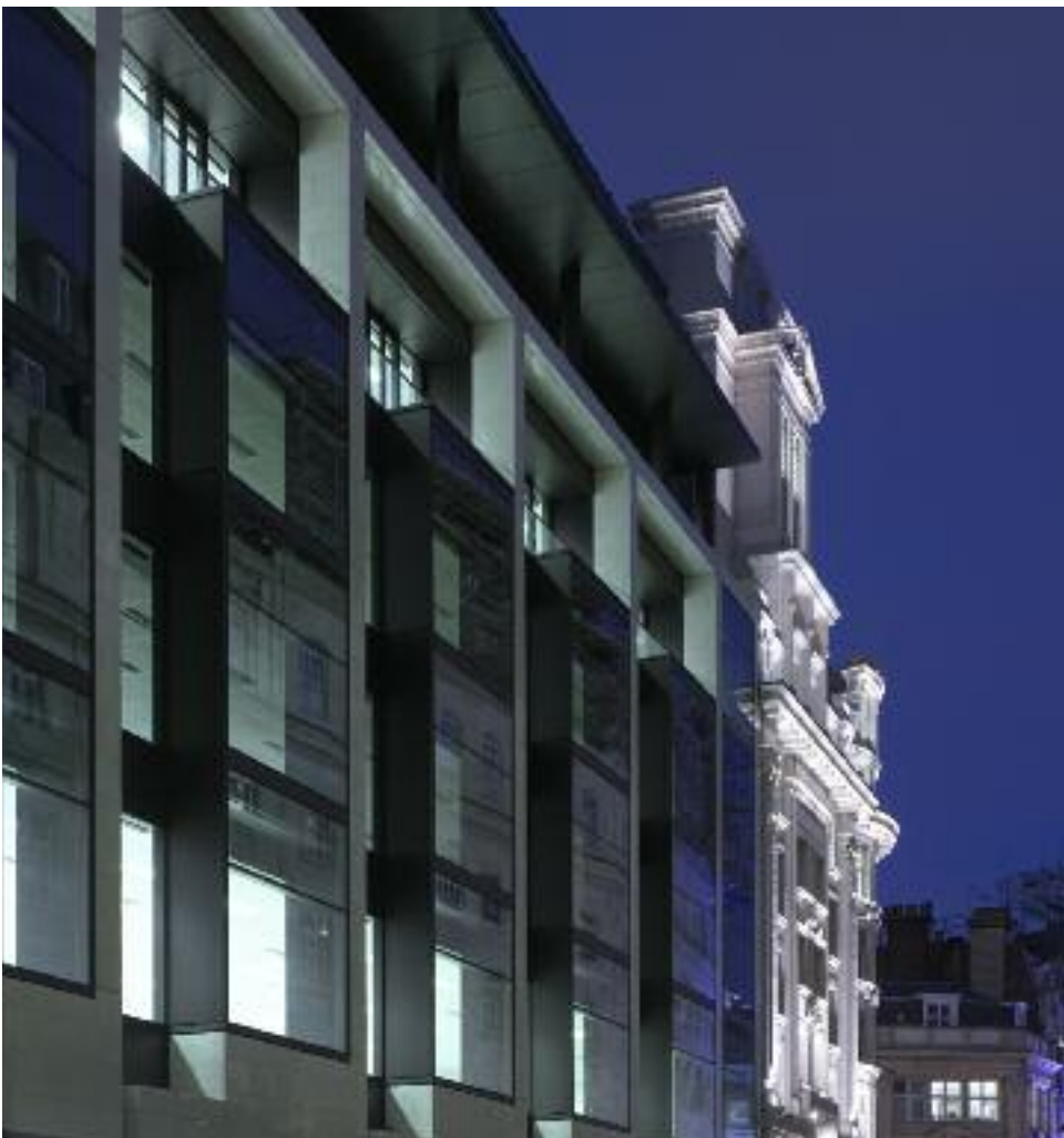
BELOW: Quadrant 3, a mixed-use development by The Crown Estate, won the Best Historic Building Management award
