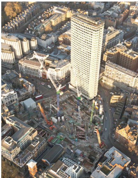
Crossrail at Centre Point
