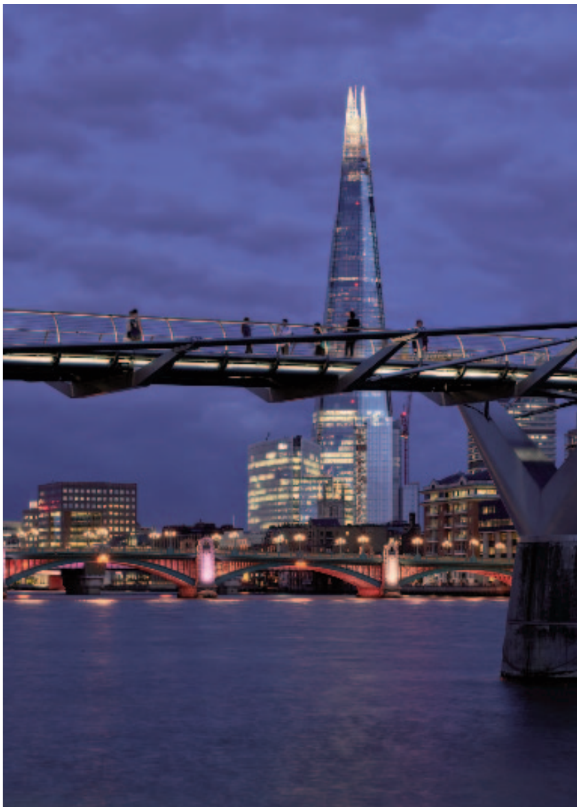
BELOW: Completed artwork on the Millennium Bridge, looking towards The Shard ©James Newton
