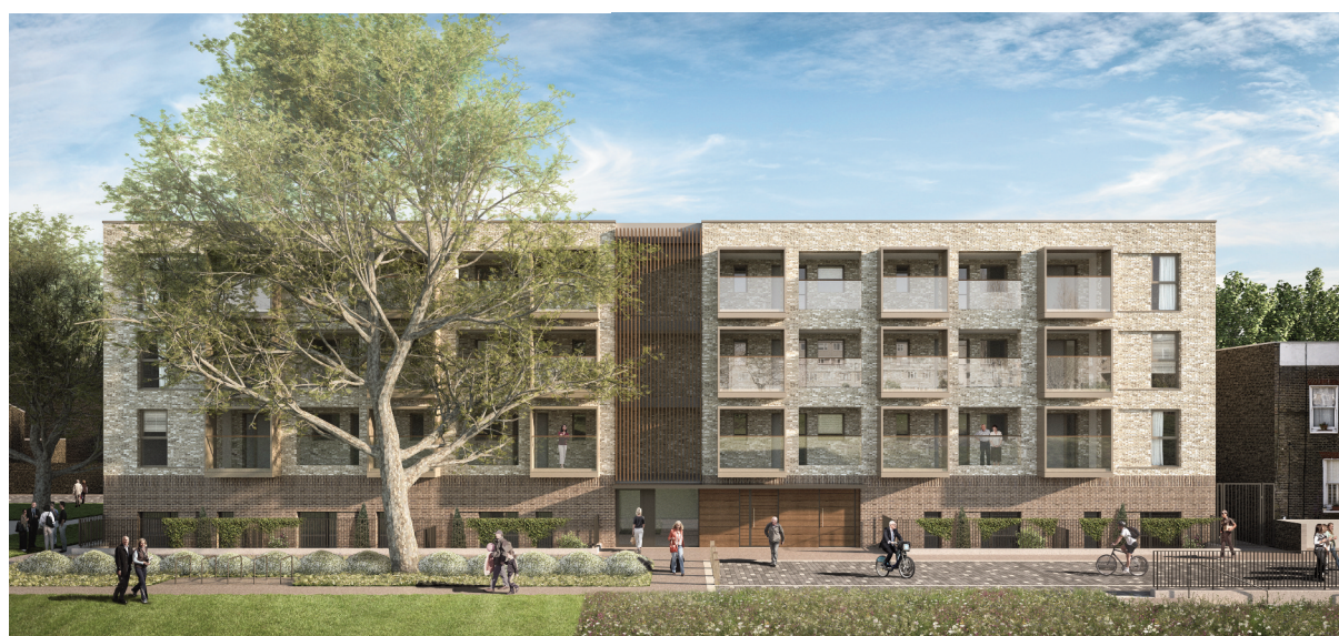
BELOW: Dover Court for London Borough of Islington
