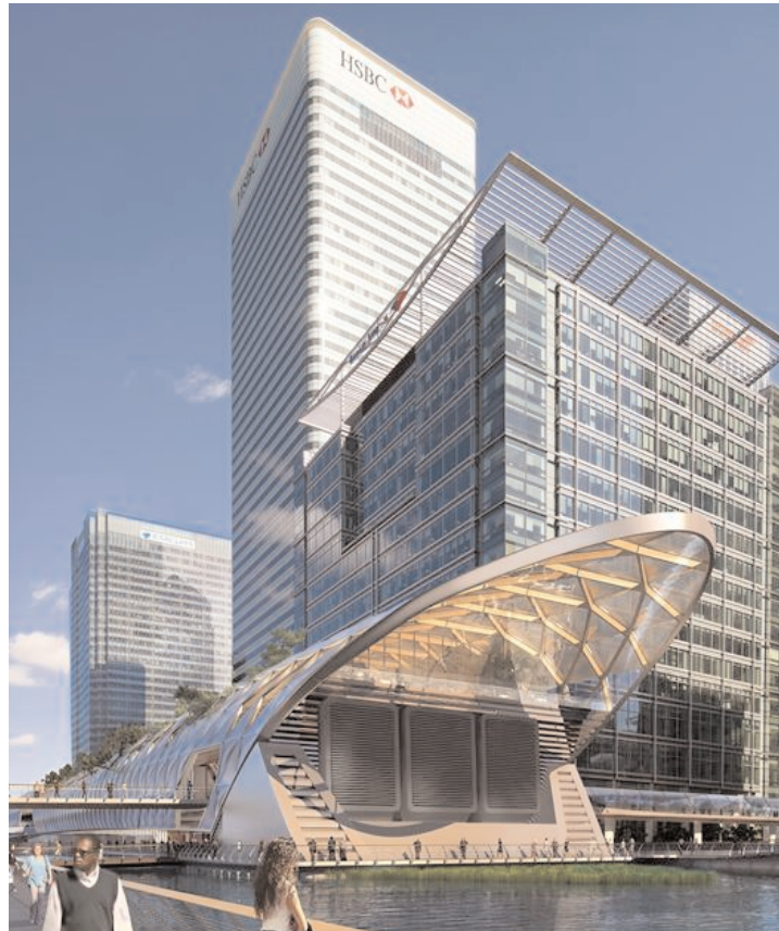
Construction got underway last month with the station at Canary Wharf
